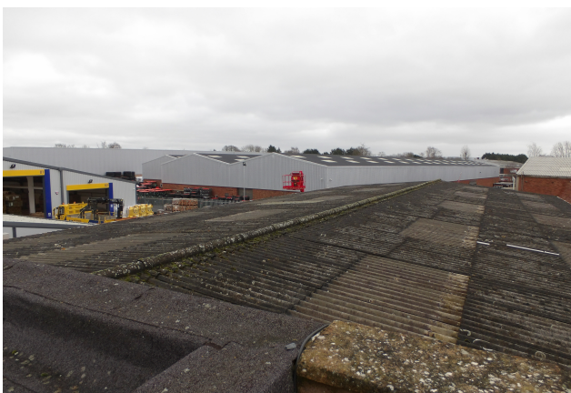
03: Profiled cement roof coverings (assumed ACM) to warehouse roof.
