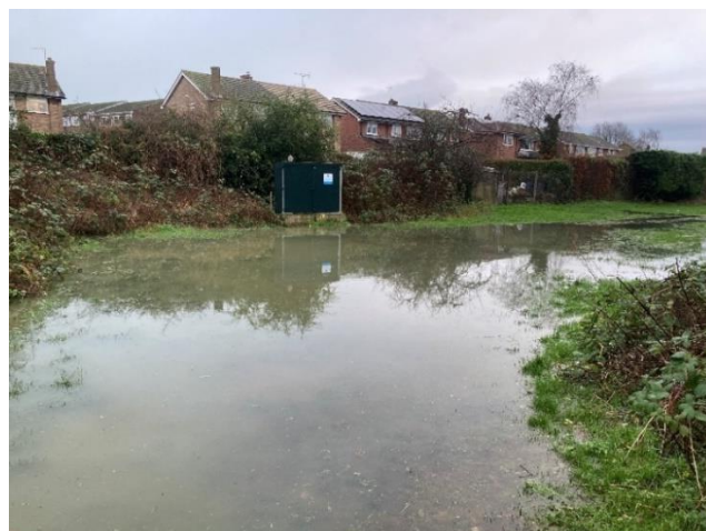
Brookside Sewage Pumping Station
