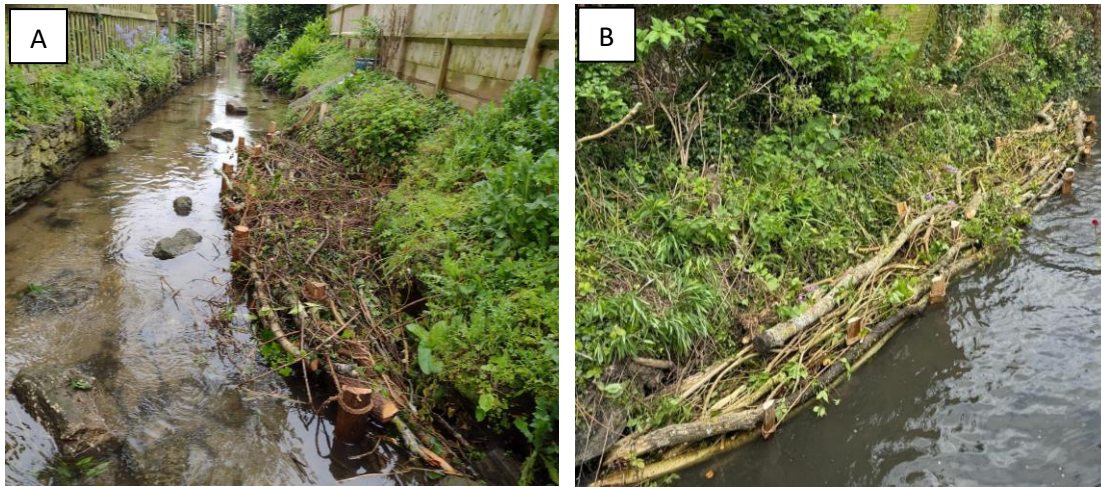
Figure 6 Photos A&B: Habitat structures constructed on the Chalgrove Brook, Chalgrove Highstreet - completed under FRAP
