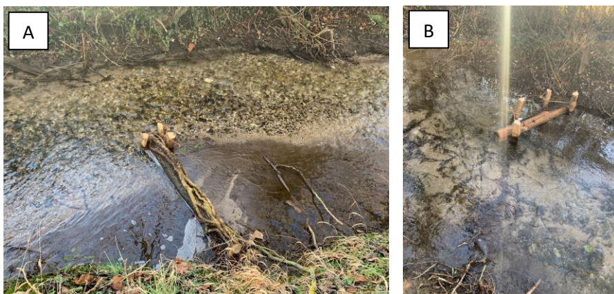
Figure 7 Photos A&B: Log features constructed on the Chalgrove Brook, Cutmill - completed under FRAP
